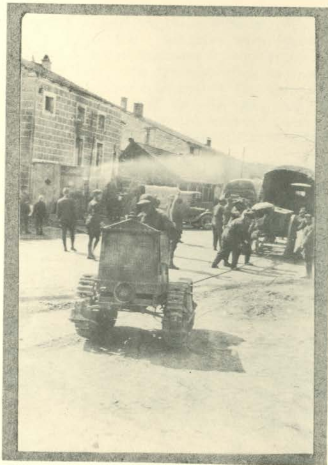
LOADING AND SUPPLY ACTIVITIES AT ENGINEER SUPPLY BASE, BLONDEFONTAINE.
