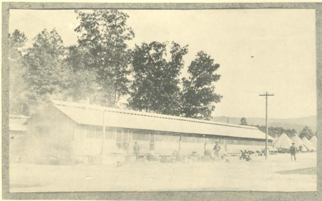
ENGINEER MESS SHACK AND KITCHEN AT HEAD OF COMPANY STREET. TYPICAL DEVELOPMENT AFTER CLEARING AREA. CAMP MC CLELLAN, ANNISTON, ALA. OCT. 1917.
