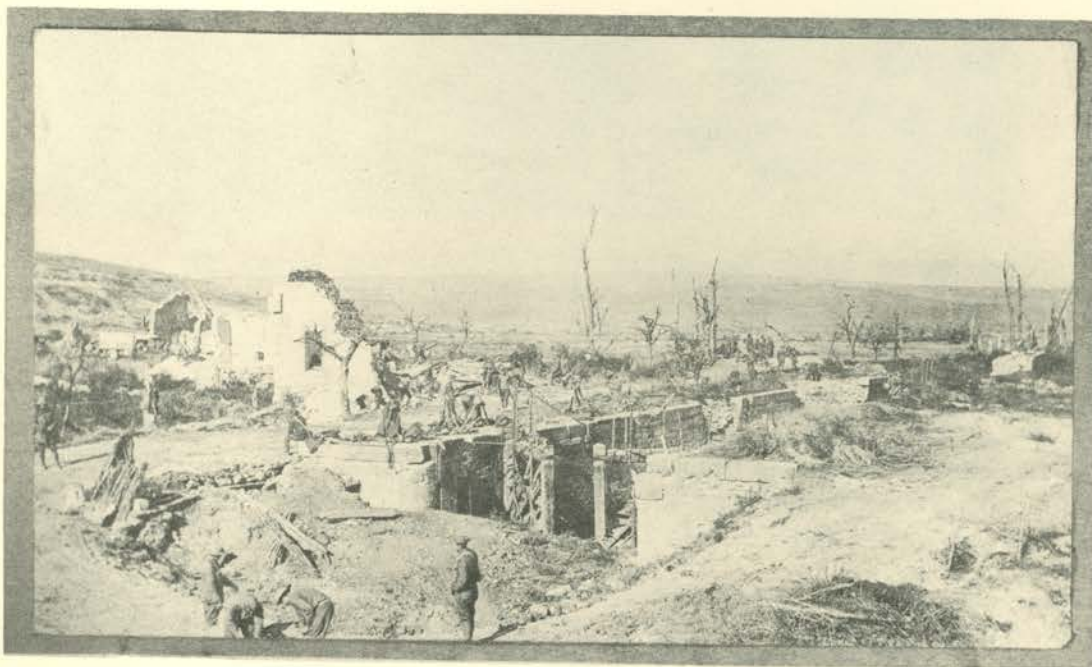
DESTROYED LOCK OF THE RHINE - RHONE CANAL NEAR FORGES. FILLED IN TO FACILITATE TRAFFIC CIRCULATION.
