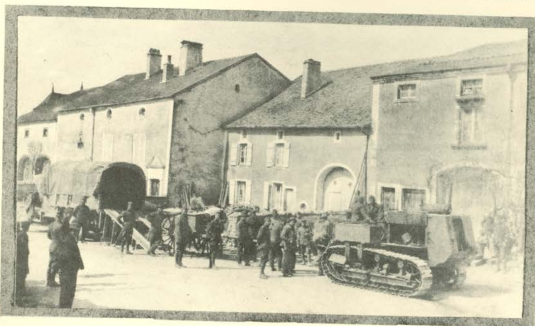
BLONDEFONTAINE, REGIMENTAL HEADQUARTERS AND SUPPLY BASE. LOADING EQUIPMENT ON TRUCKS IN PREPARATION FOR MOVEMENT BACK TO COAST AND EMBARKATION FOR HOME.
