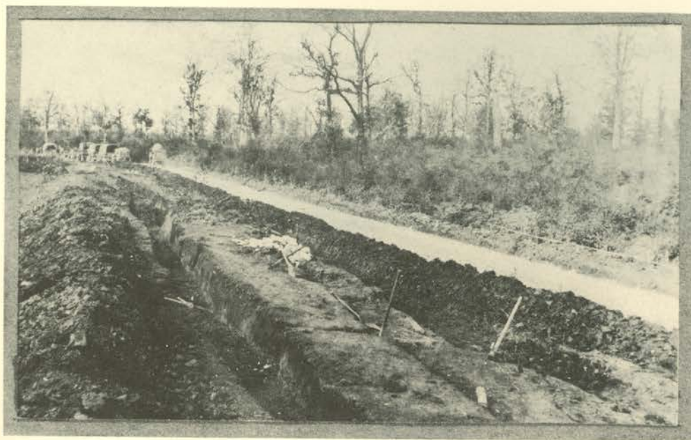
ROAD FROM AVOCOURT TO CHEPPE. REPAIRED WITH BARE HANDS DURING NIGHT TO MOVE ARTILLERY INTO POSITION THEN ENTIRELY RECONSTRUCTED WHEN EQUIPMENT COULD GET THROUGH.
