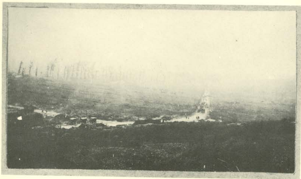
ALL THAT REMAINED OF SAMOGNEUX AFTER BUILDING MATERIAL HAD BEEN USED FOR ROAD REPAIR.
