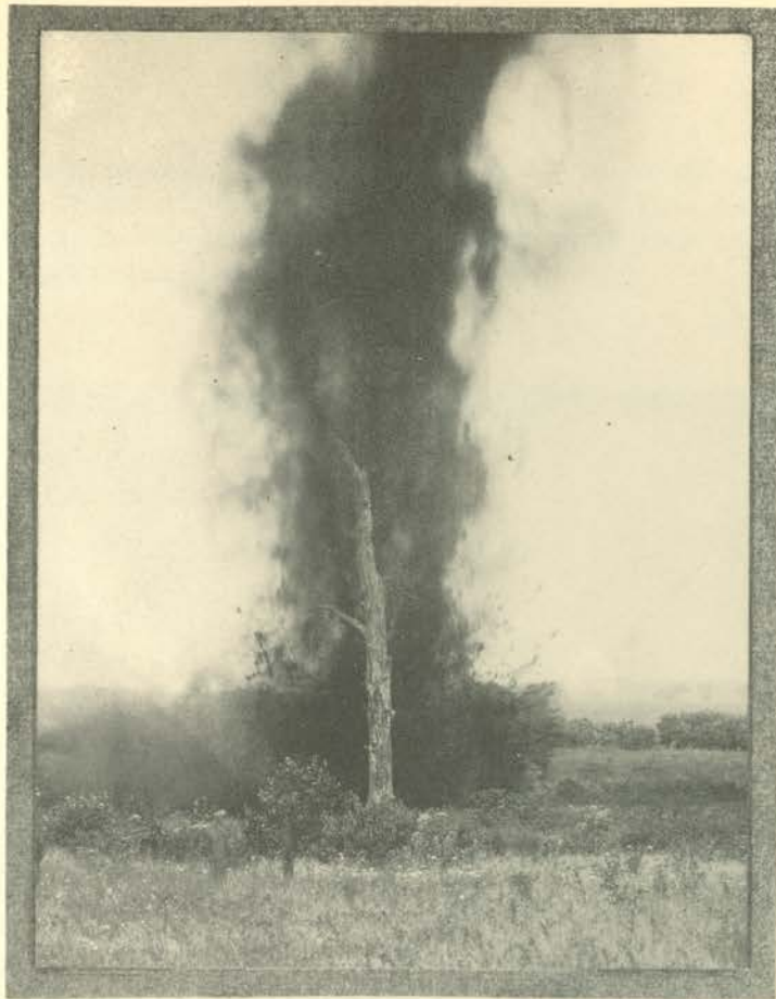
ENGINEER OPERATIONS AT GREGORY FARM. DEMOLITION DETAILS CLEARING STREAM BED.
