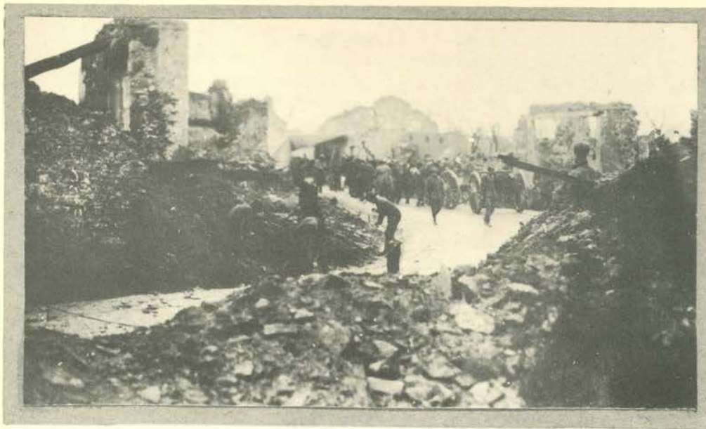
CLEARING THE ROADS AND PULLING DOWN TOTTERING WALLS IN FORGES.
