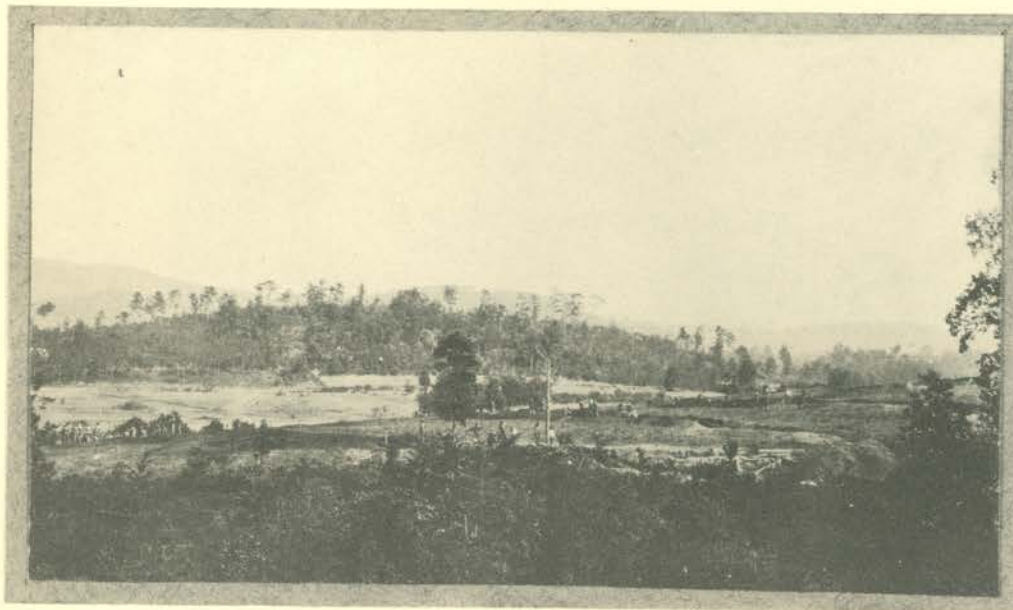
TRENCH AREA DEVELOPMENT, CAMP MC CLELLAN, ANNISTON, ALA. OCTOBER 1917.
