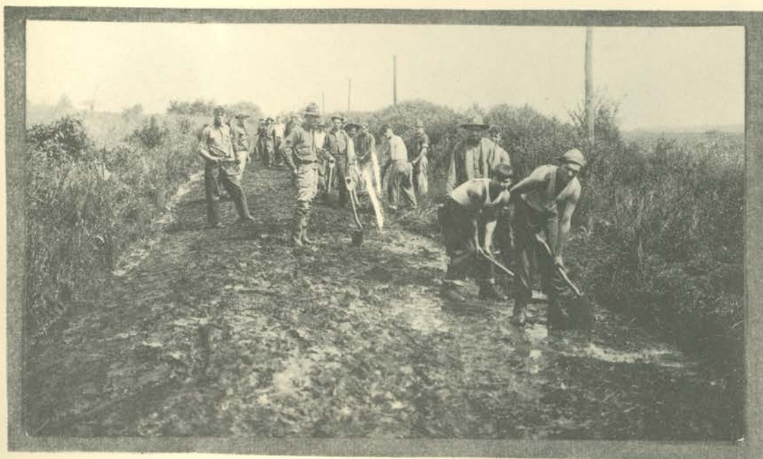
ENGINEER OPERATIONS AT GREGORY FARM. ROAD REPAIR AND DRAINAGE.
