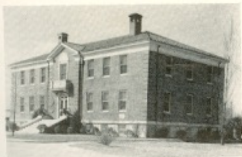
Field Artillery Board Building.
