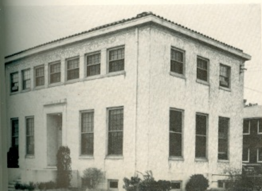
POST SIGNAL OFFICE
